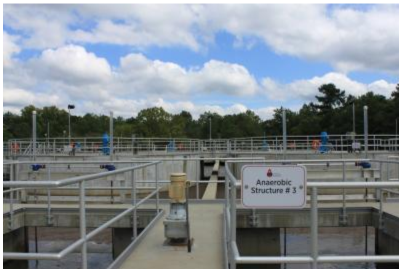
Figure 1 City of Dallas WWTP
