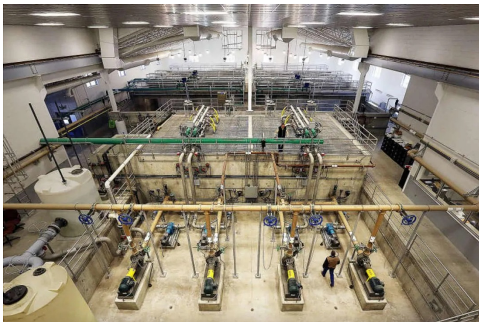
Figure 1: Inside the Jordanelle MBR Facility
