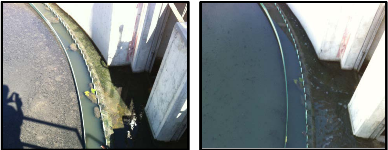
Figure 3. Secondary clarifier before (left) and after (right) introduction of RE100
